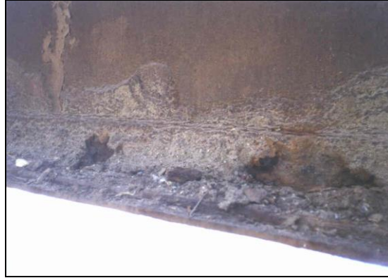
Figure 28. Photo. Heavy corrosion of bottom flange and web due to collection of poulitce.
