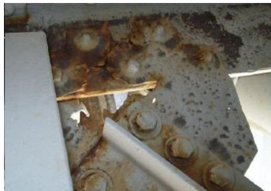
Figure 38. Photo. Corroded lateral gusset plate detail.
